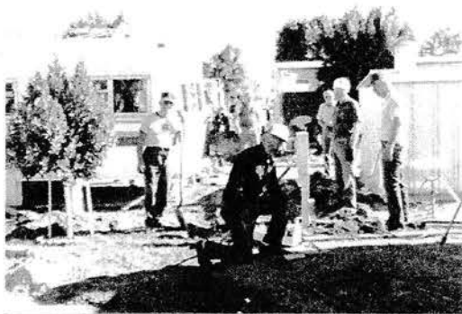
Repairing Damage To Electric Lines Caused by Moles—1986
